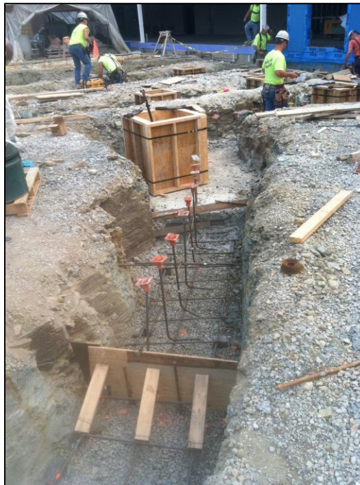
Figure 1: Construction of Chapel Footers & Column Piers (Property of Mascaro Construction)
