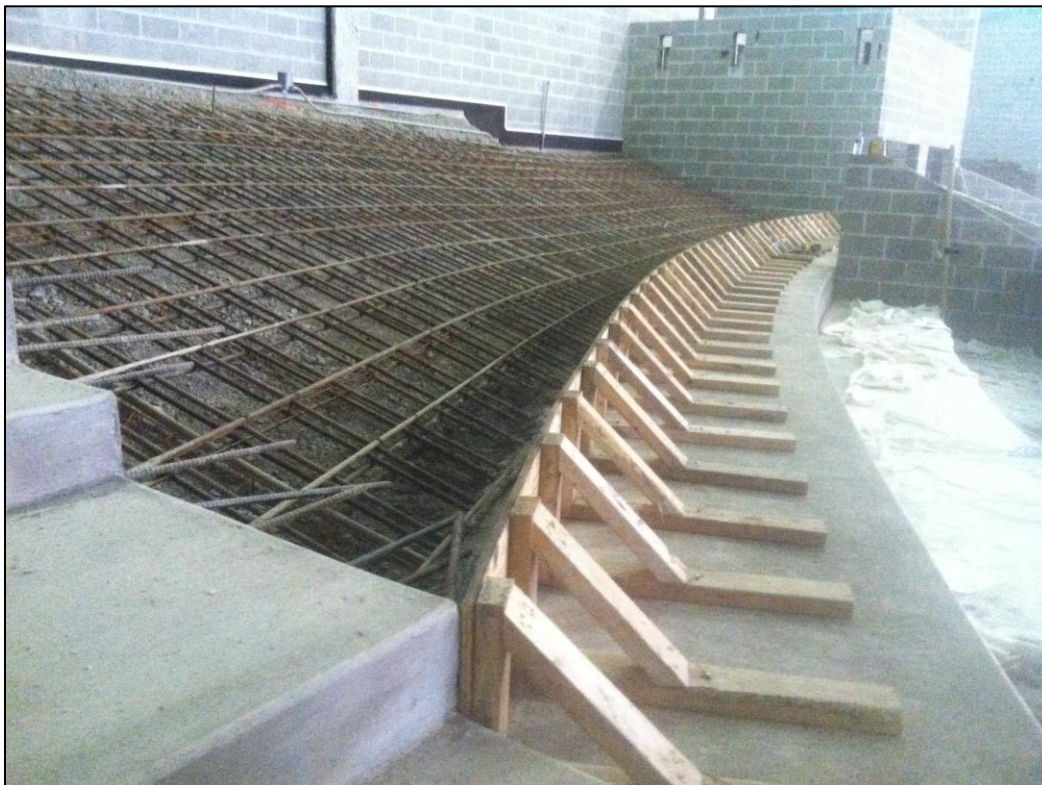
Figure 4: Auditorium Riser Seating Construction (Property of Mascaro Construction)
