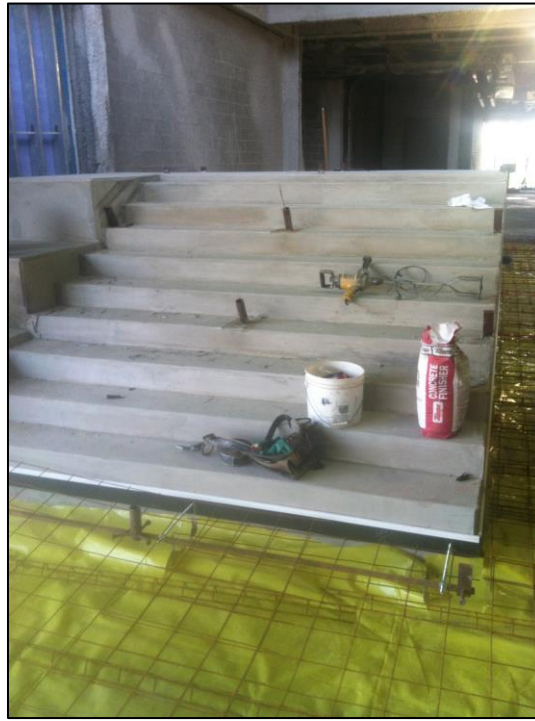
Figure 7: Recently Poured & Finished F11 Staircase (Property of Mascaro Construction)
